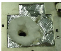
Figure 3.12. Cut into the Insulation
